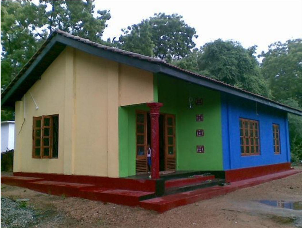
The completed school room.
