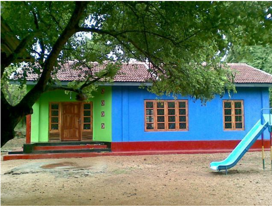
The school room is brightly colored and an attractive addition to this community.
